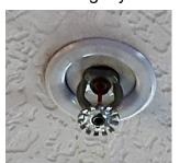
Figure 87-Fire Sprinkler Head
