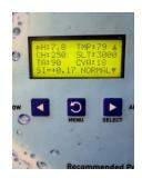
Figure 96-Pool Chemistry Controller
