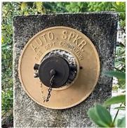
Figure 86-Dry Hydrant Connect
