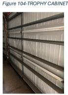
Figure 107-Hurricane reenforcing bars
